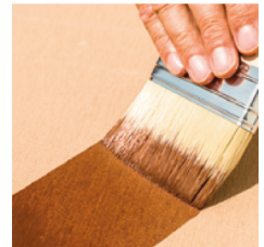
STAIN OR PAINT
